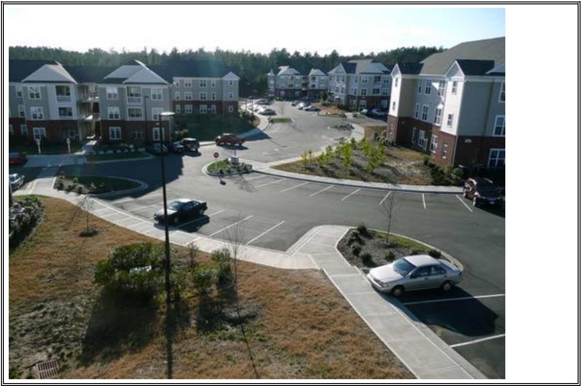
Photograph Number 3: Typical Subject Property interior view – note asphalt and flatwork in good condition
