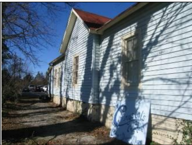
9. Building 113 left side or south elevation – pier and curtain wall foundations
