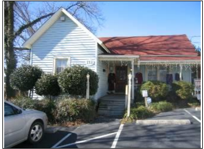
8. Building 113 front/east elevation at Main Street
