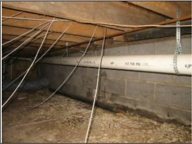
55. Structural view 3: no cracking observed at Building 115 crawlspace
