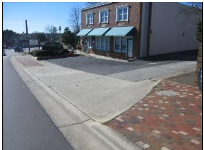
22. Concrete apron at Building 115 access from Main Street
