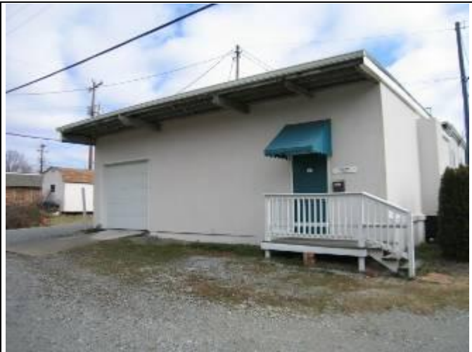
5. Building 115 rear or west elevation – unit D
