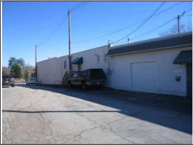
7. Building 115 north elevation – paint warehouse and unit A
