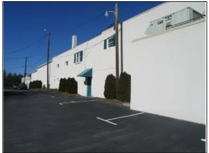
4. Building 115 south elevation – Stucco finish
