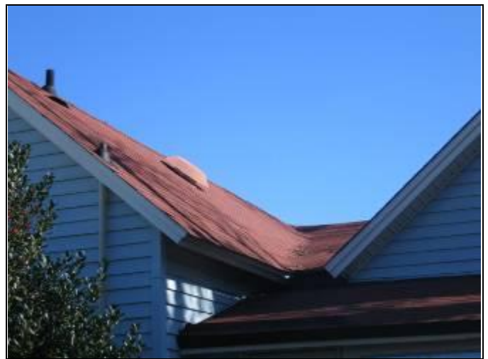
34. Building 113 rear roof view showing waste vent flashings and no gutters
