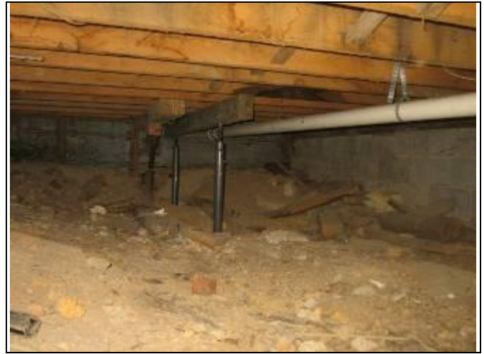
56. Structural view 4: Screw-jacks with drop-girders provide additional floor bracing crawlspace bldg 115
