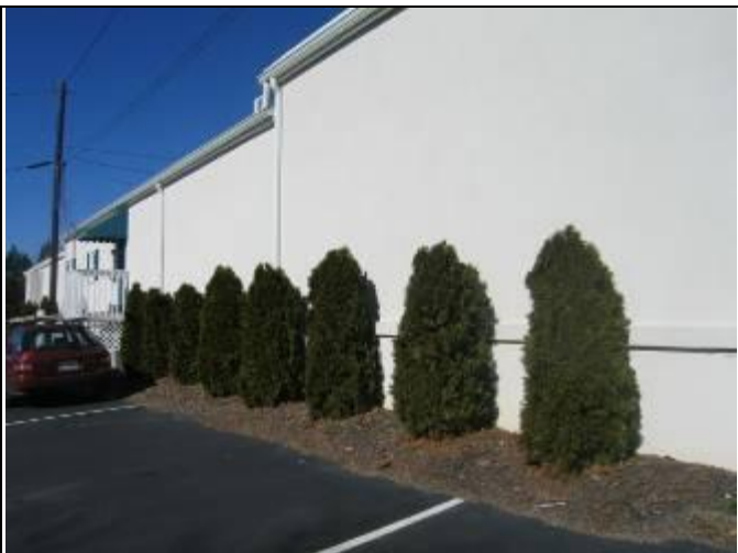
53. Structural view 1: significant cracking in exterior walls not observed at Building 115
