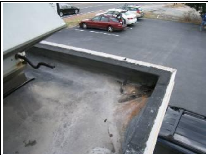
27. EPDM membrane over Building 115 unit A public toilets
