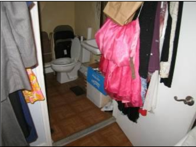
73. ADA accessibility view 3: Building 113 toilet not configured for wheelchair traffic and cannot be without expensive renovations
