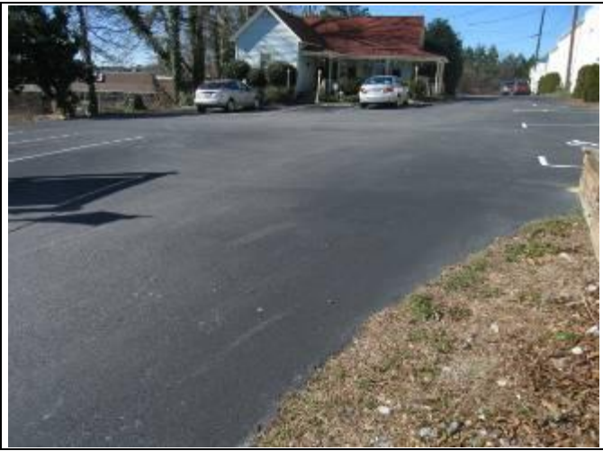
13. Asphalt access drive to building 113 and 115 parking
