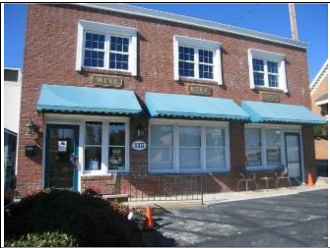
3. Building 115 east elevation
