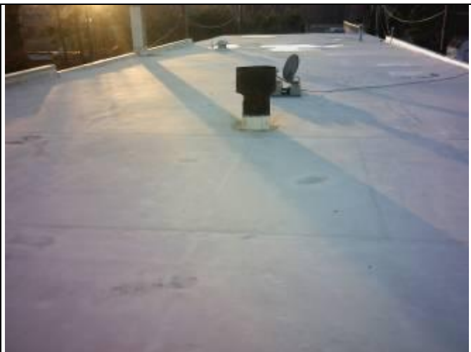
23. TPO roof membrane view west – area of possible moisture in foreground
