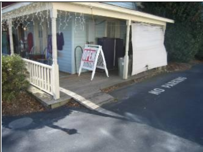
11. Building 113 north elevation porch, access ramp and heavy shrubs
