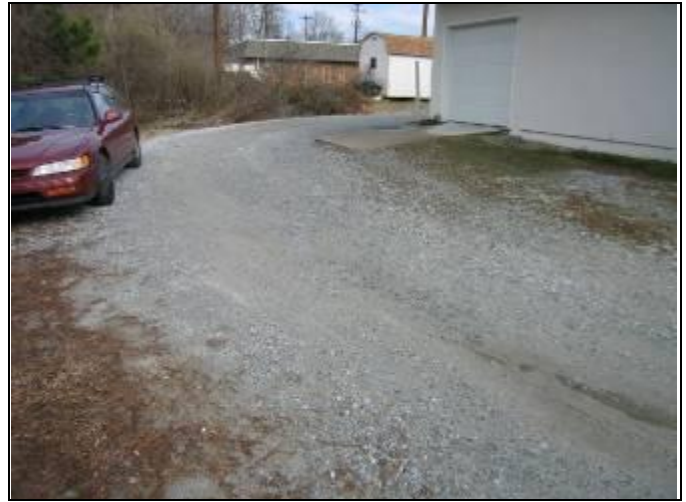
20. Number 20: Gravel drive behind Building 115
