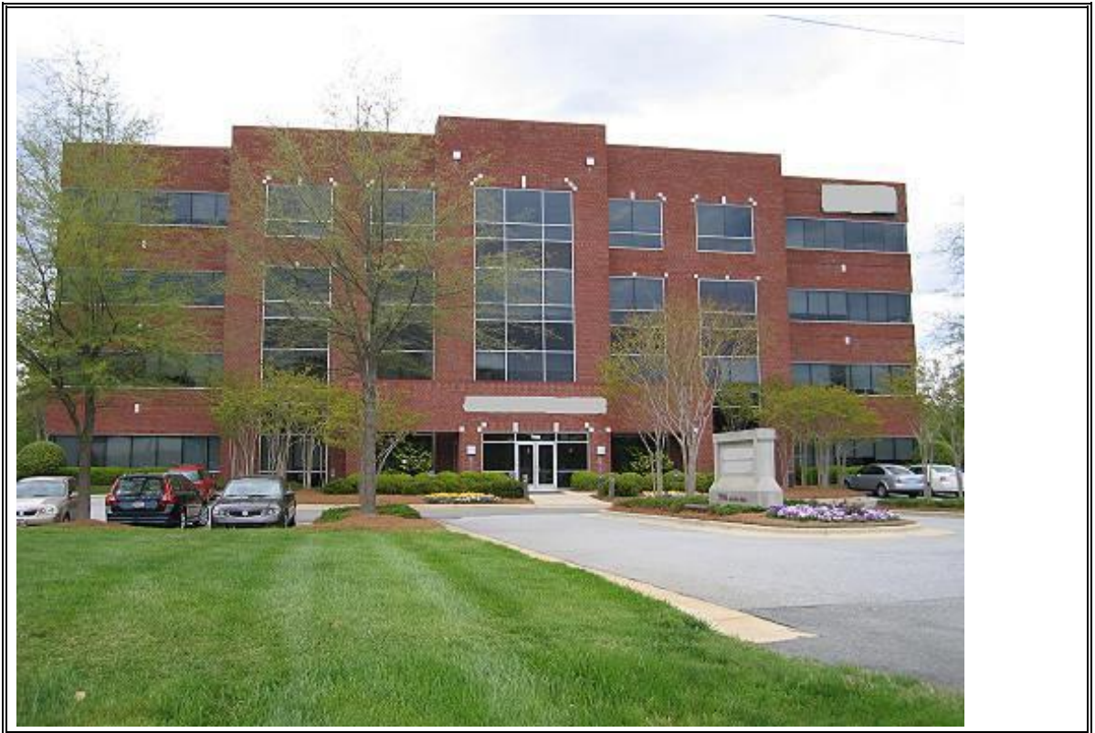
Photograph Number 1: Subject building entry driveway at Business Park Blvd
