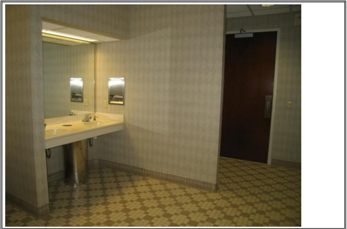
Photograph Number 7: Typical ADA accessible toilet area
