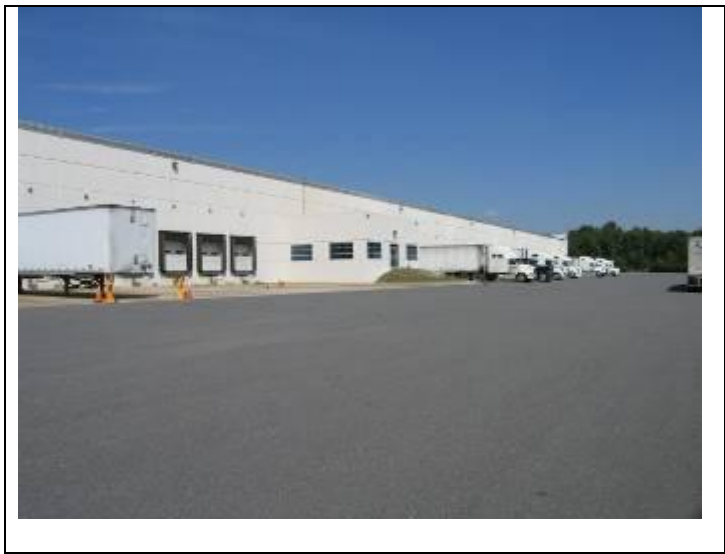
8. East elevation loading areas and asphalt condition
