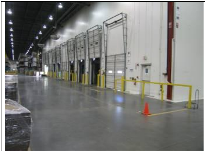
33. Interior loading area
