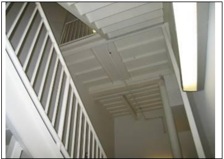
20. Metal framed interior stairwell in good condition
