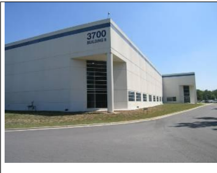
1. Subject Building main entry at Widget Drive –
