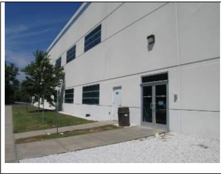
7. Employee entrance - typical tilt-up-wall construction
