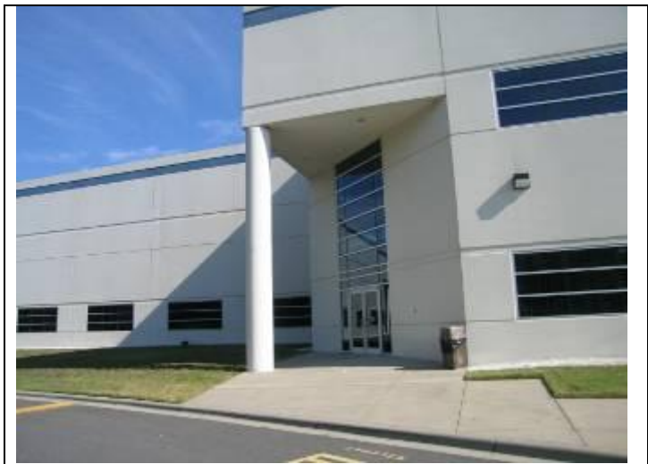
12. One of two main entries with store-front hardware
