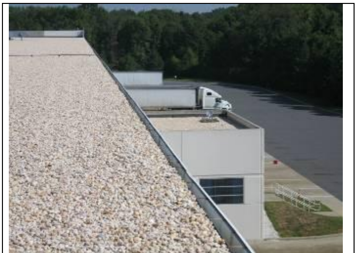
40. Ancillary rooftop over shipping/receiving office – ballasted membrane
