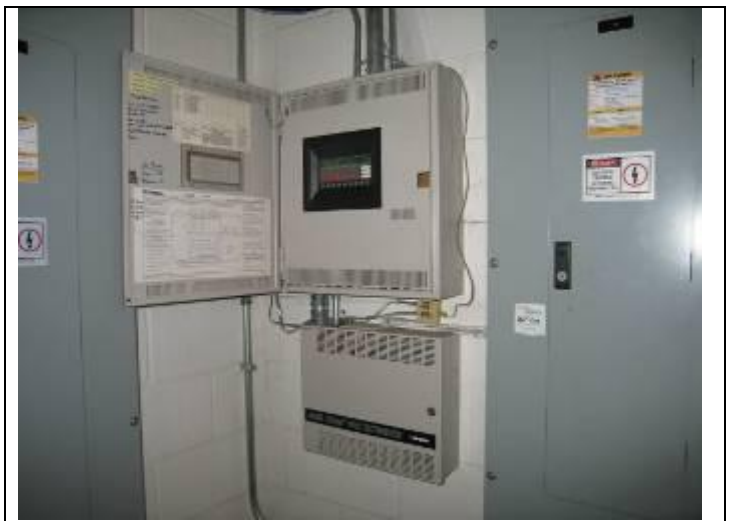
30. Monitored fire alarm system in switchgear room
