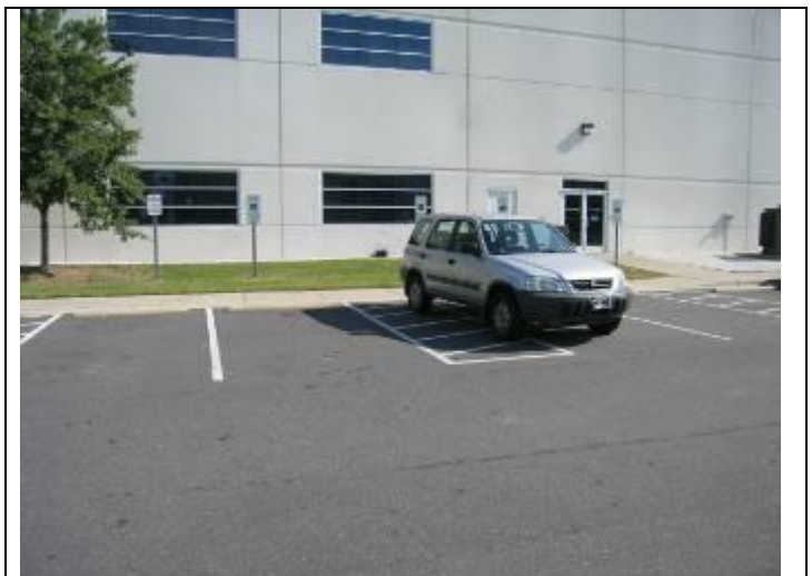
4. ADA parking spaces (five total) - van accessible
