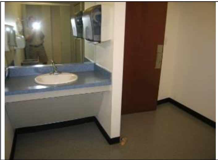
15. Office area ADA accessible toilet
