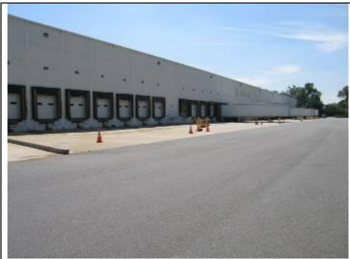
11. West elevation loading area and driveways
