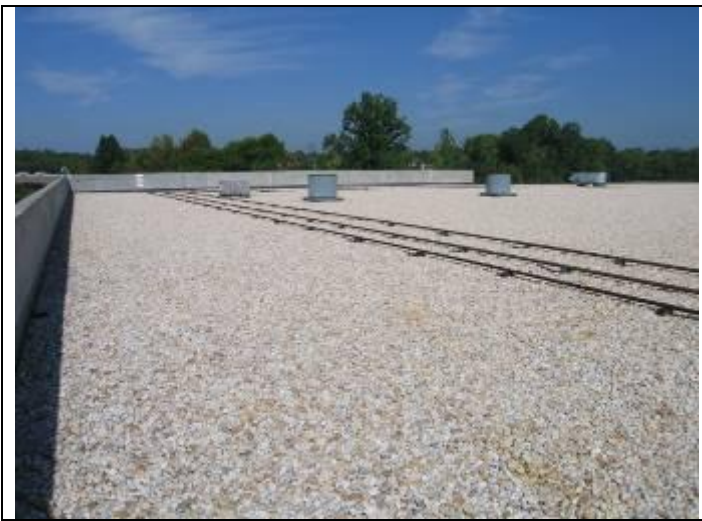
37. Natural gas distribution piping, typical ventilation fans, Gravel ballasted EPDM roof membrane
