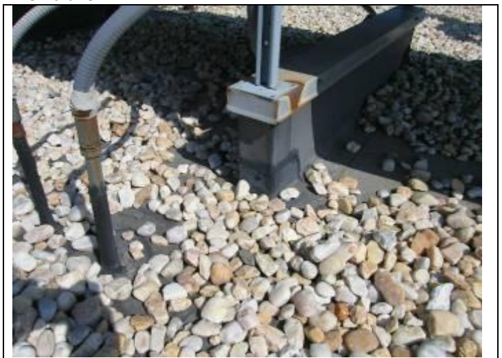
42. Flashing detail - prior repair evident
