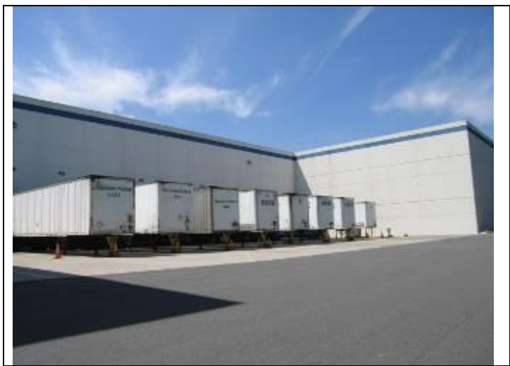
10. Subject Building North elevation loading area
