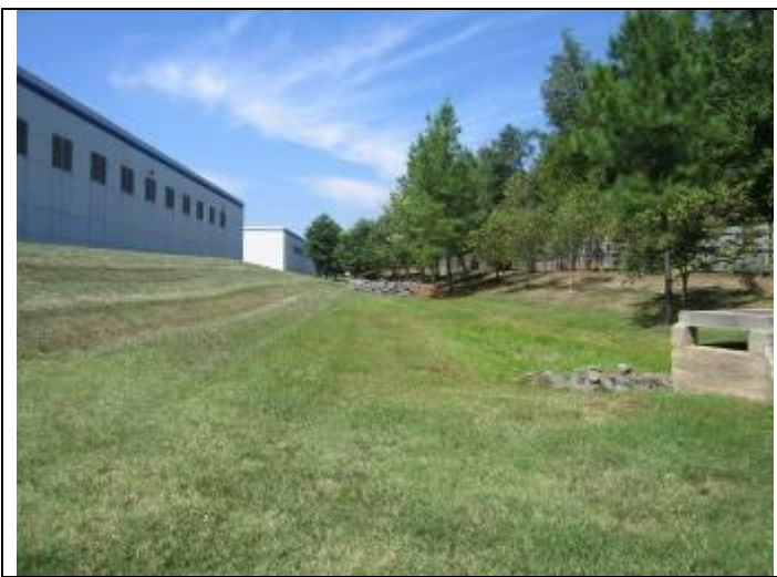
9. Building North elevation and run-off/retention area
