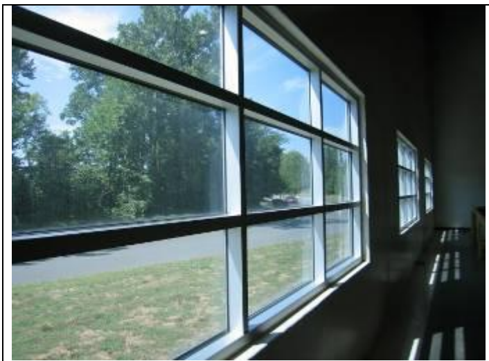
35. Extruded aluminum framed insulating glass windows
