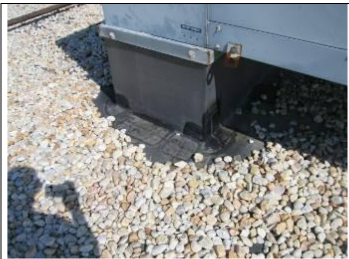
41. Flashing repair to single membrane rubber at RTU
