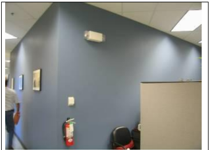
18. Current fire extinguisher, emergency lighting
