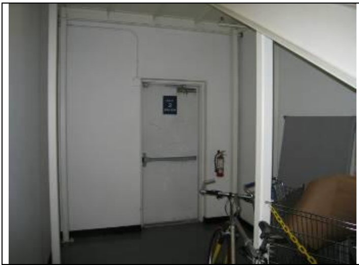
19. Stairwell and exterior door, current fire extinguisher
