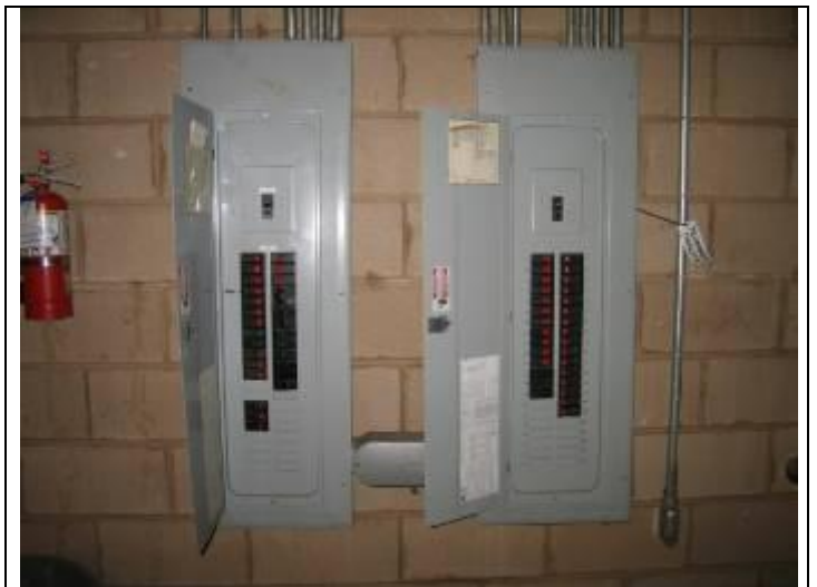
42. Twin main service panels at Wilbur's Widget Mfg. with 200 ampere maximum buss ratings per panel and 225 ampere main breakers installed.
