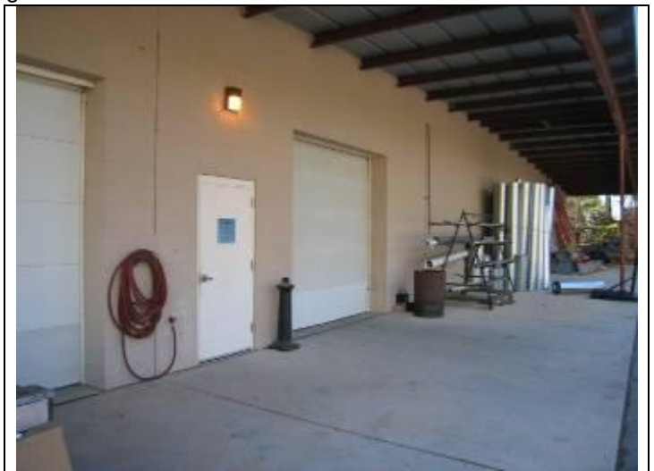
10. Rear service doors in good condition – typical exterior lighting
