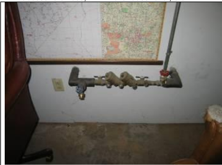
41. Water supply shut-off with back flow prevention
