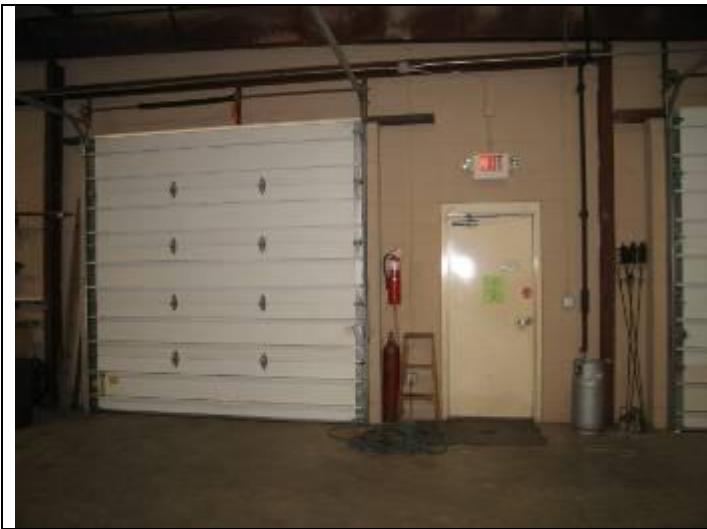
33. Warehouse/loading bay and rear service doors – fire extinguisher current
