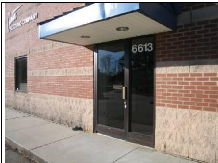
13. Front entry with storefront style doorframes with full height glass insulating panels (one of two)
