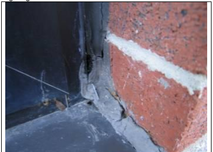
12. Damaged caulk will permit stormwater to wall interior cavity
