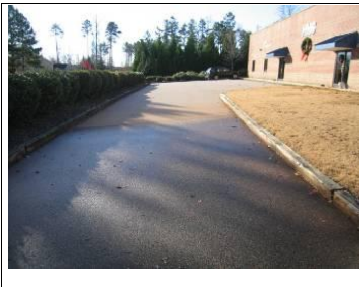
7. Asphalt front drive lane and parking – wood curbing
