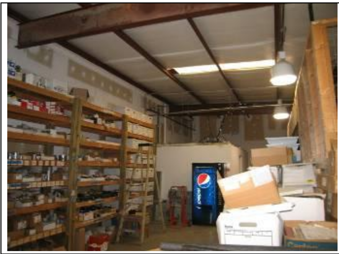
25. Canter Electric storage area adjacent to south elevation wall
