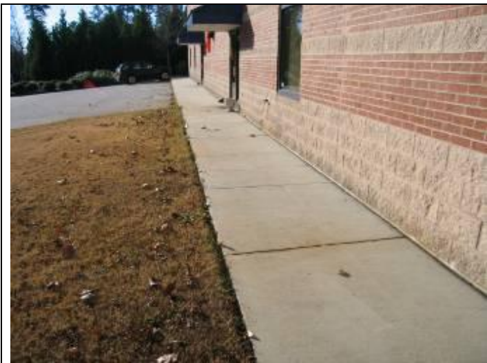
9. Front walkway typical of good flatwork condition
