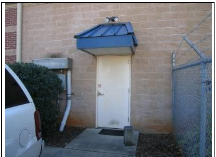
14. North side service entrance adjacent to utility meters (electric and gas)
