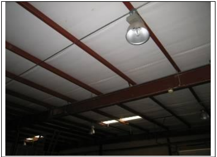
34. Warehouse area steel framing and HID lighting – insulated roof deck
