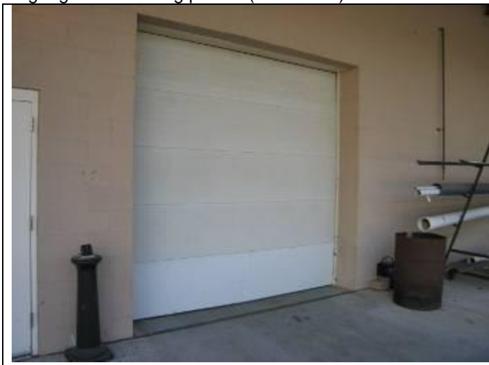
15. Rear loading area sectional door in good condition
