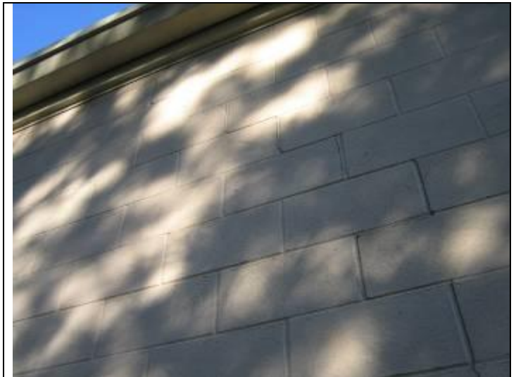
24. Through-block and stair-step cracking at south elevation
