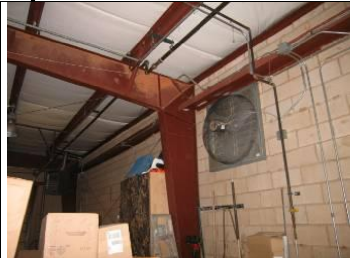
35. Warehouse area steel framing detail and exhaust fan at north wall
