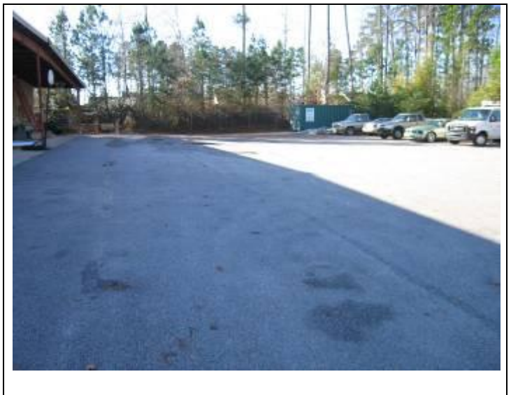
8. Rear service/staging area with asphalt paving in typical good to fair condition
