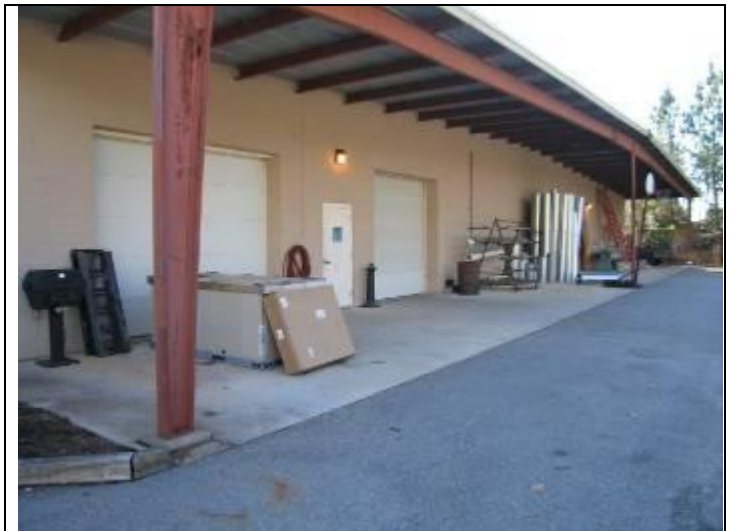
4. Rear (west) elevation and loading/service areas
