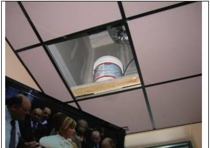
28. Reported (2) roof leaks bldg 5954 - 170 (area one of two)
