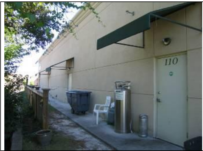
19. Rear elevation Building 5916 and unit 110 MB's Grille
