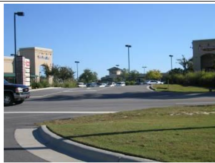
1. Subject Property main entry at Sanders Road
