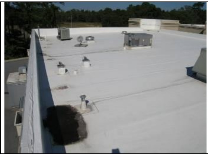
43. Building 5920 above units 140, 160, 170 single membrane
