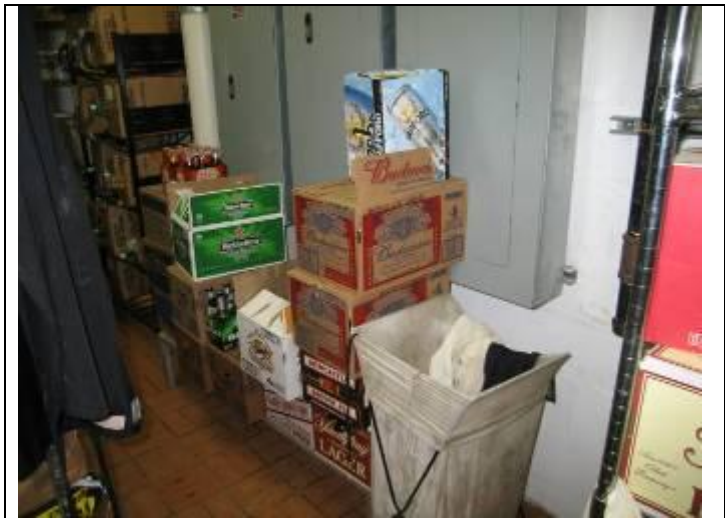
24. Blocked access to switchgear at rear of HoBoy Steakhouse
