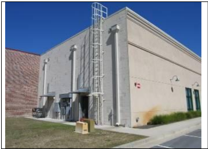
14. Bldg 5920 units 110,120 – Sprinkler riser room inaccessible
