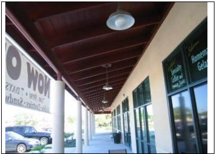
8. Exposed walkway framing & lighting typical for Property
