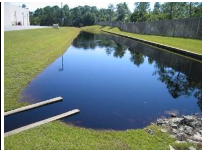
15. Retention pond system continues west/behind building 5920
