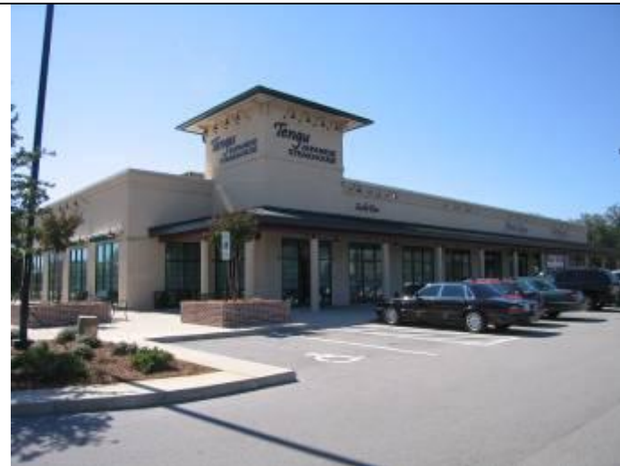
5. Building 5954 and typical ADA Van accessible parking
