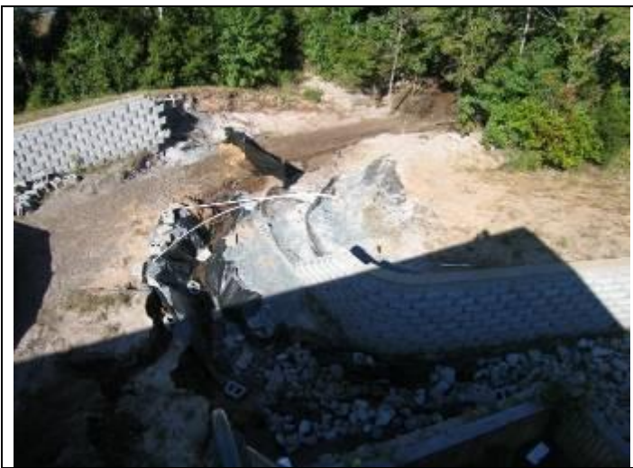
21. Roof view incomplete retention pond behind bldg 5916
