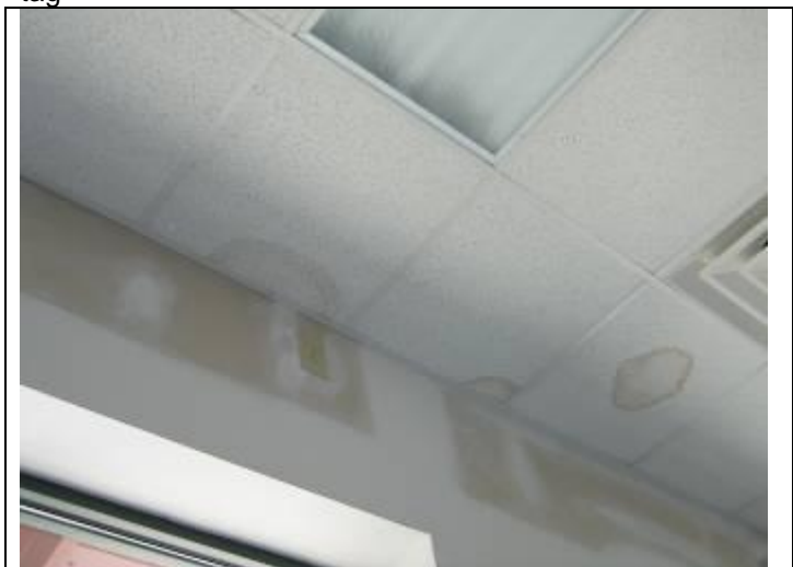
36. Building 5916 vacant unit 130 with suspect ceiling stains
