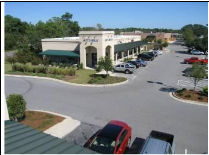
17. Rooftop view Building 5916 – typical site landscaping
