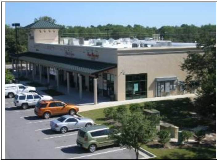
7. Roof view bldg 5954 typical unit electric utility metering
