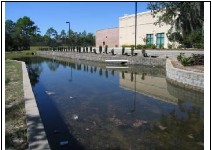
10. Retention pond system continues west of Building 5954
