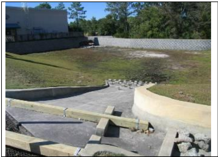
20. Site view of incomplete retention pond east of bldg 5916
