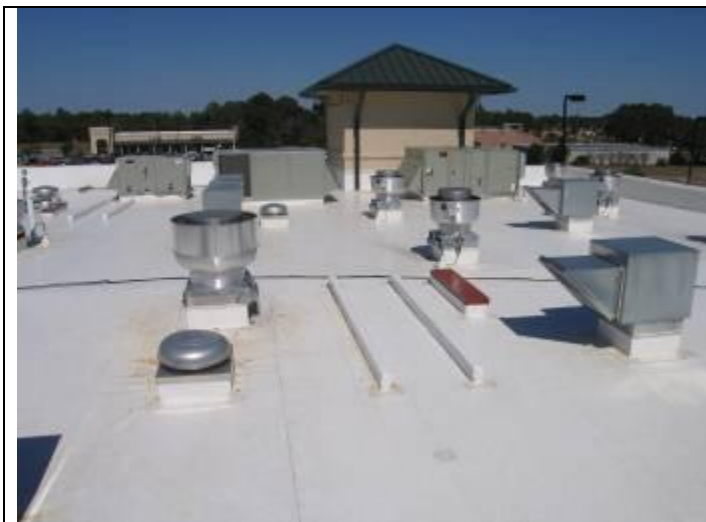
41. Building 5954 above Unit 110 HoBoy Steakhouse
